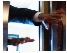
ScanGUARD® provides 63 non-parallel infrared beam paths with a range of 0-6 ft. (0- 1.83 m).
