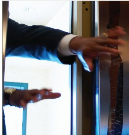
ScanGUARD® provides 63 non-parallel infrared beam paths with a range of 0-6 ft. (0-1.83 m).
