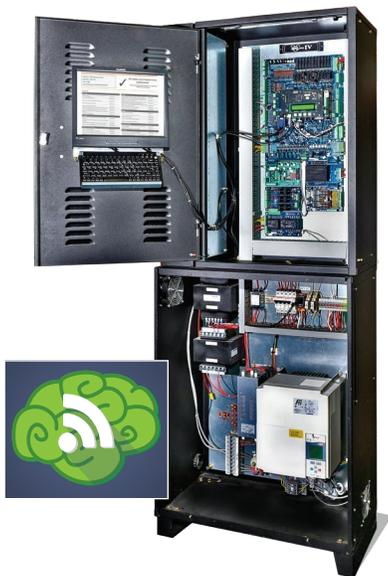
*GALaxy IV's secure built-in Wi-Fi capability offers a smarter way to access a complete library inside, and the ability to upload a completed MCP and archive it within the Controller for future review.*
