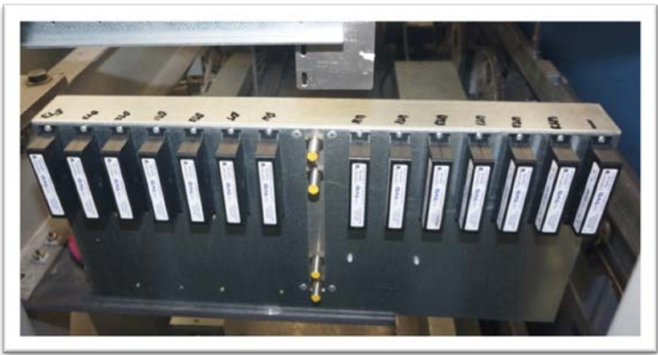
Figure 2.10: Typical Selector Box Installation
