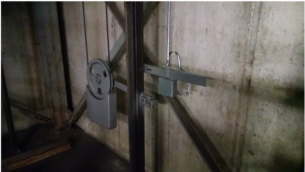
Figure 2.15: Bottom Bracket Mounting
