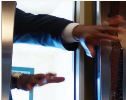
*ScanGUARD® provides 63 non-parallel infrared beam paths with a range of 0-6 ft. (0- 1.83 m).*
