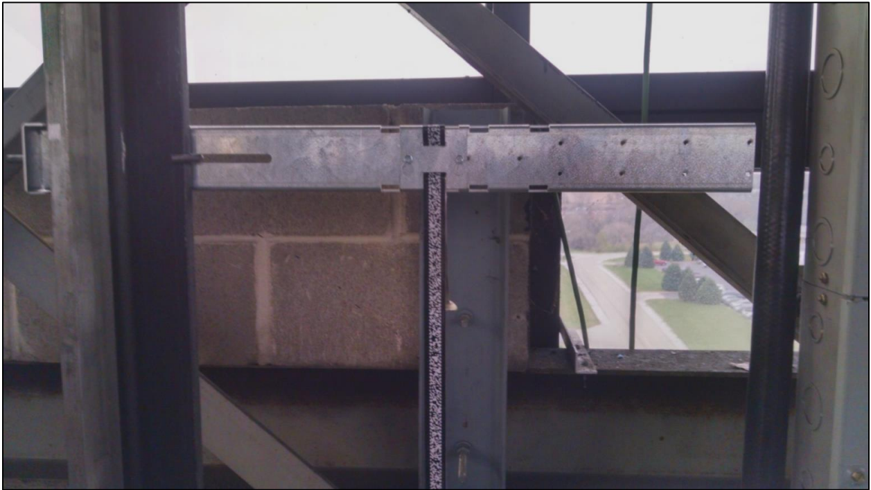
Figure 2-1: Encoded Tape Mounting – Top Bracket
