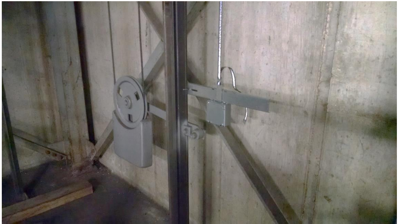
Figure 2-8: Encoded Tape Mounting – Bottom Bracket
