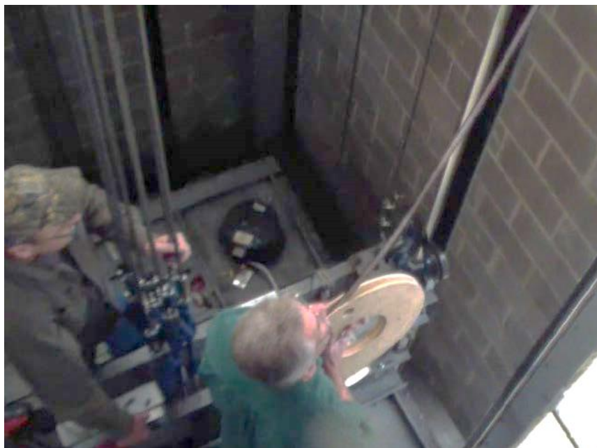
Figure 2-5: Unroll the Encoded Tape
